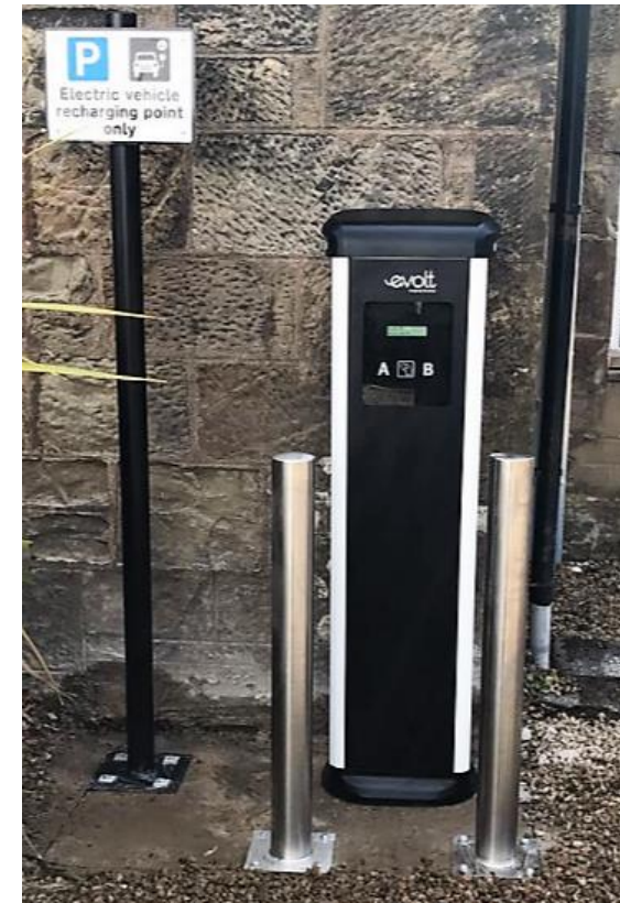
Example of Post eVolve installed next to a wall
